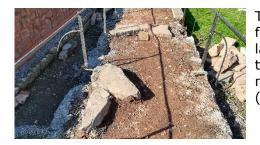
The existing edging stones are in Lias, as are fragments of paving that can still be seen under the layer of bitumen macadam at the far south end of the footbridge. When we peeled back the bitumen macadam, we found further evidence of Lias slabbing (as shown in the picture).
