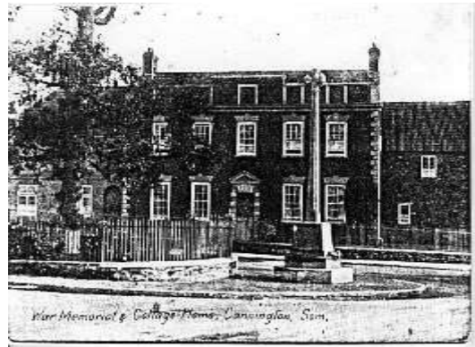
Old postcard showing original location of War Memorial and adjacent railed garden. The memorial was moved forward during the construction of Hinkley Point 'A' power station.
